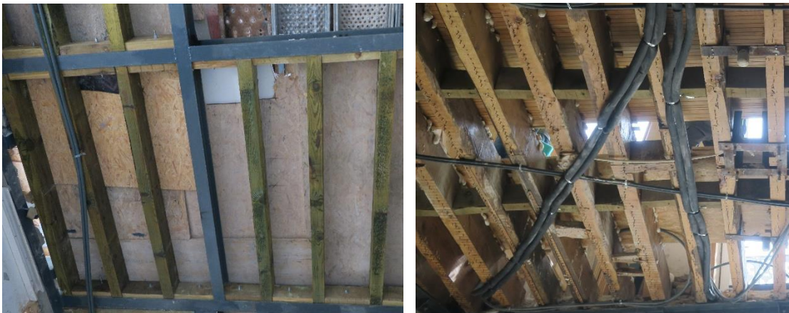
Figure 5.1 - Photography of intervention in timber pavements in Palacete Faria
